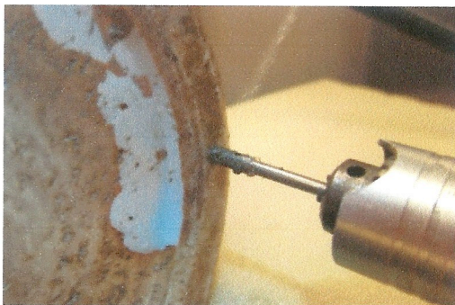
Water is used during drilling to prevent heating. 進行核心取樣時以冷水降溫。
